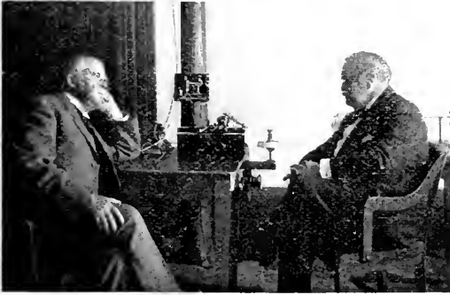
Inventor Delany and Chief Engineer Larish reading from a Telepost Instrument which has been "slowed down" to a speed to permit reading by sound.
